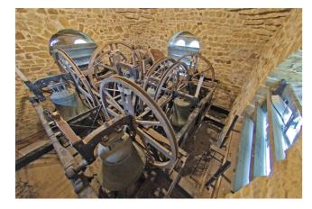
The whole restoration project involves removing the two oldest bells through the roof of the nave, casting two new bells and hanging them. Other necessary work includes replacing the headstocks on the two largest bells, cleaning out and possibly replacing the main bearings, regrinding the clapper balls to restore their shape, repairing and rustproofing the metal bell frame, replacing the pulleys, repairing the stays and hanging the two old bells separately beside the bell frame.
